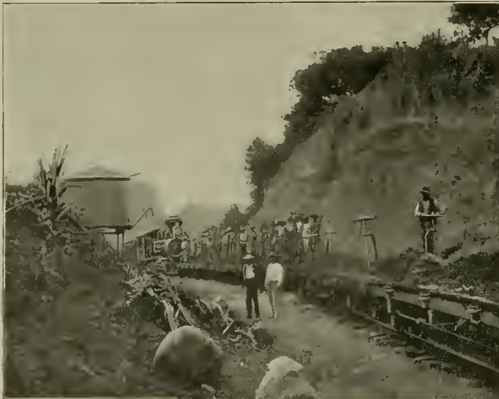
WORK TRAIN, SANTA ANA RAILROAD.
